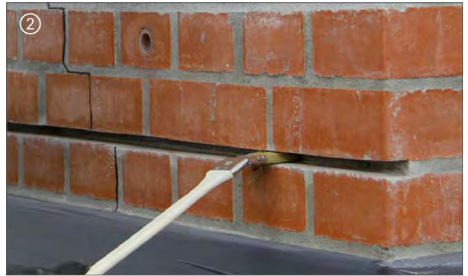
Fuge reinigen | Nettoyer le joint
